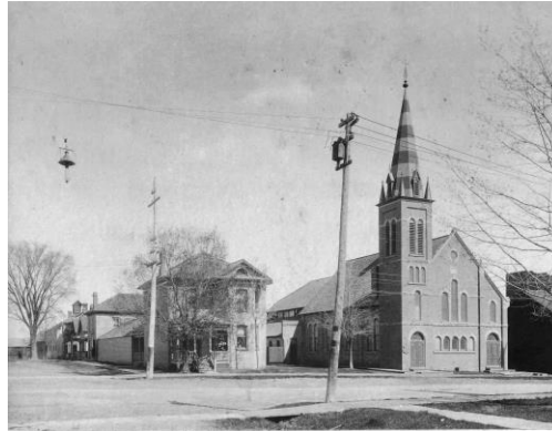
Brick parsonage on corner built following the fire of 1895. Drive sheds rebuilt behind. It is interesting to note the tree down the left hand side where the post office street is now.
